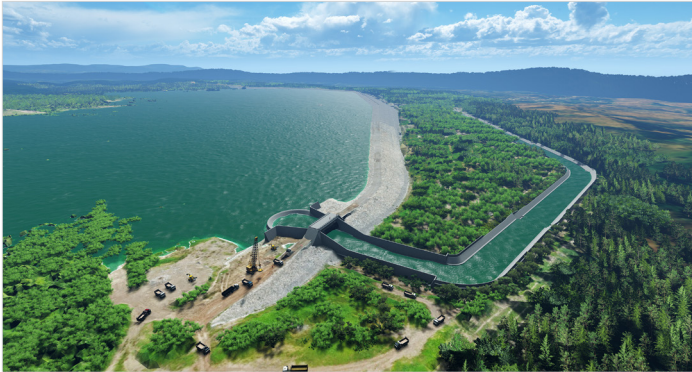
Adjusting the slope design to ensure strength and safety helped the organization avoid an estimated USD 1.8 million in rework while ensuring continued safety. Image courtesy of PT Hutama Karya (Persero).
