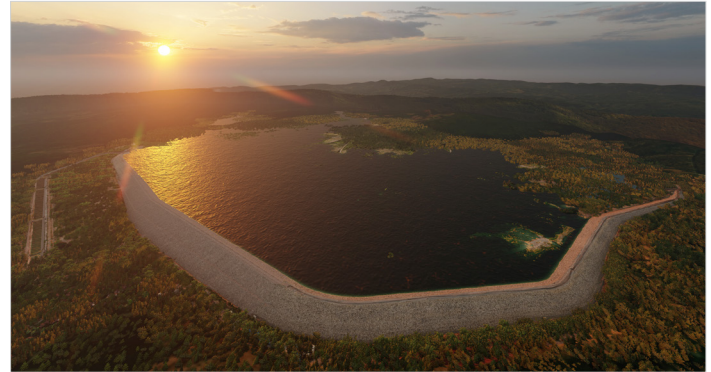
Geotechnical analysis eliminated the need to construct a grouting foundation and reconstruct the secant pile, saving USD 2 million. Image courtesy of PT Hutama Karya (Persero).
